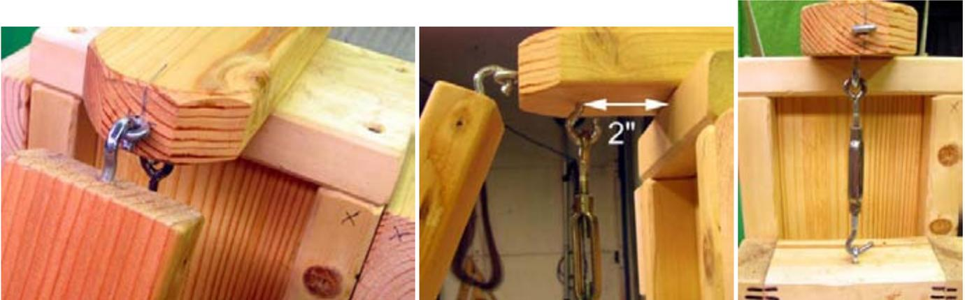
**Clearance:** Part K is adjusted for a close clearance but not touching either the grinding head or the front side of the grinding cup. The same clearance is required for the exit chute (P).
